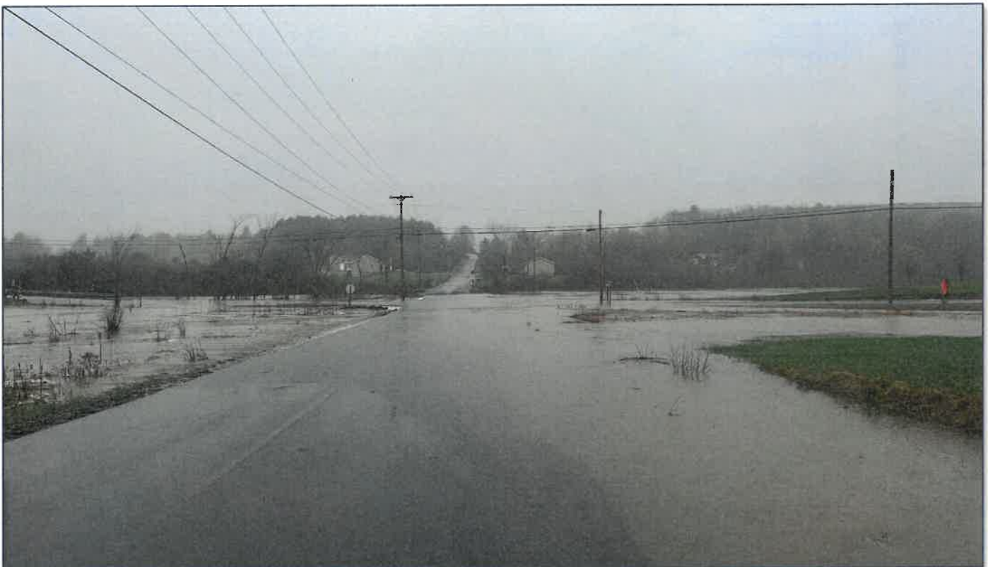
Intersection of East Rd and Avenue Rd, Wales ME, Road flooding. Source: Wales Fire Chief Scott Dimmick.
